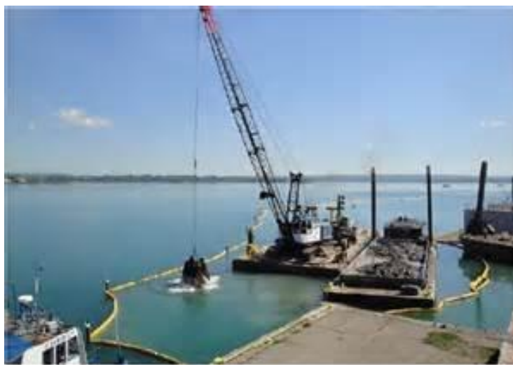
Figure 4. Photograph of Mechanical Dredging
