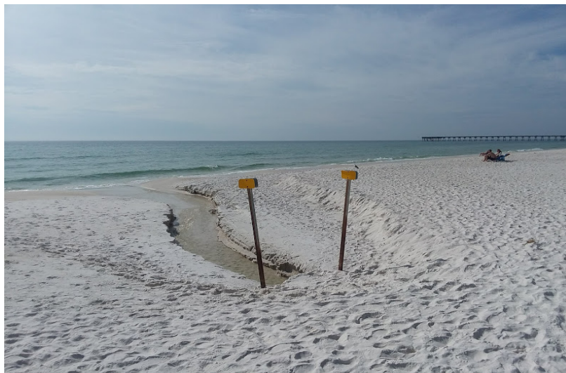
Fig. 1 Non-extended outfall on a nourished beach
