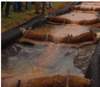
Figure 1. Examples of sediment control BMPs: (a) Coir Wattles treated with Polyacrylamide installed in a ditch line used to reduce velocity and turbidity of water and (b) hydroseeding with a mixture of site-specific PAM, native warm season grass seed, rye grain, hydromulch, and slow release fertilizer.
