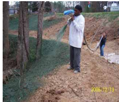
Figure 1. Examples of sediment control BMPs: (a) Coir Wattles treated with Polyacrylamide installed in a ditch line used to reduce velocity and turbidity of water and (b) hydroseeding with a mixture of site-specific PAM, native warm season grass seed, rye grain, hydromulch, and slow release fertilizer.
